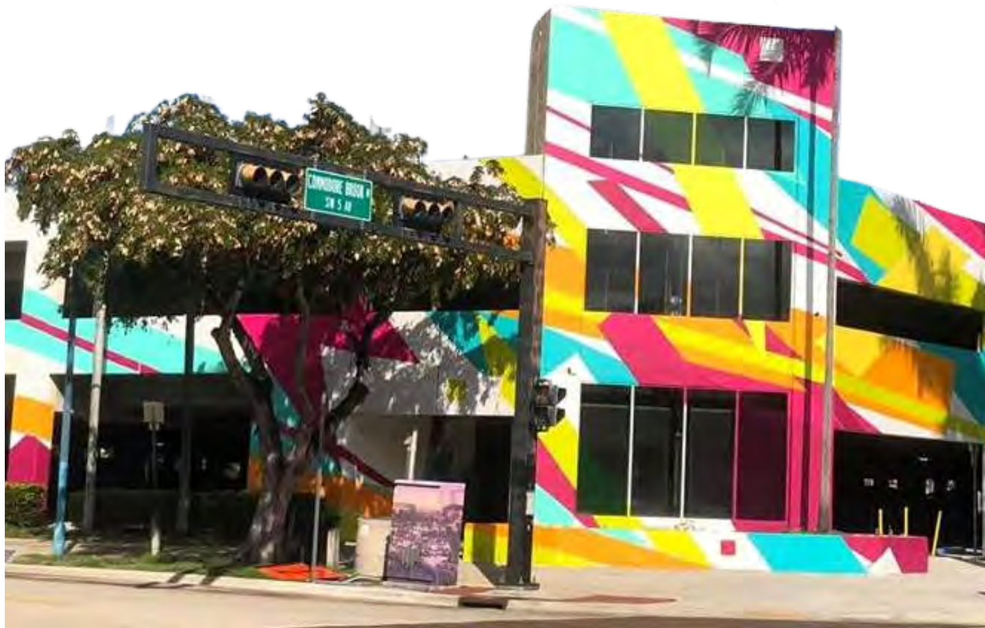
Across the street parking garage
